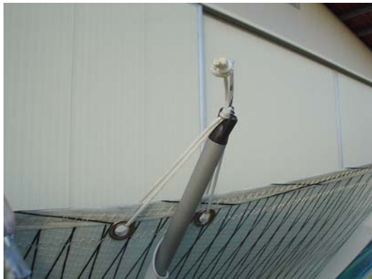
Detailed photo of properly attached batten tie.
